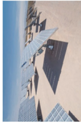
Amonix Dual Axis Concentrated PV 1.2 MW
