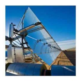
Parabolic Trough Collector
