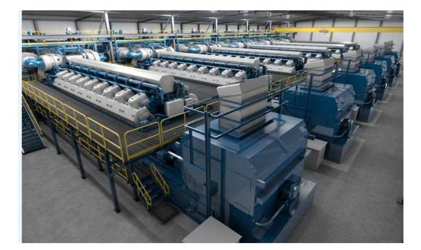
Figure 34 - Reciprocating Internal Combustion Engine Facility
