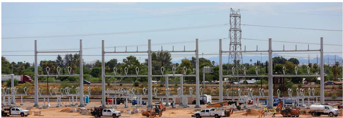
TEP is upgrading the Irvington Substation to accommodate new generating resources.
