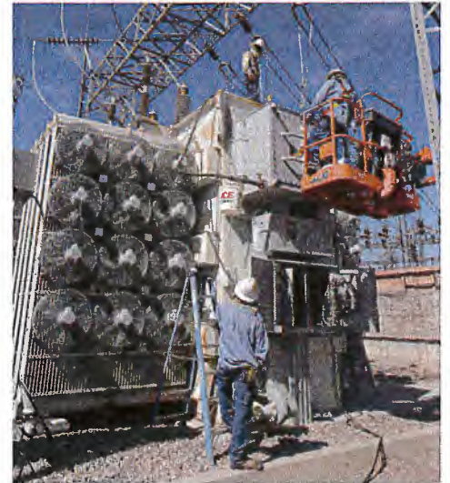
TEP employees install upgrades at the East Loop substation. The planned transmission line would connect East Loop to new and existing substations.
