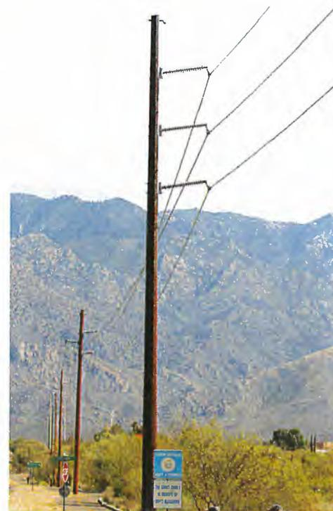
*A typical weathering steel monopole supporting a 138 kilovolt transmission line.*
