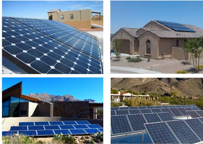
Picture 1 – Typical Residential Distributed PV Systems
