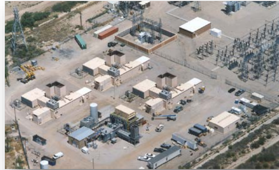
North Loop Generating Station
